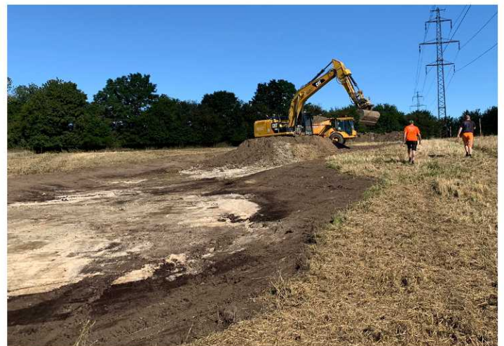
Figure 6. Construction of the lowland in september 2020. The nutrient-rich top soil is removed to expose the underlying nutrient-poor sandy soil which will encourage biodiverse vegetation.
