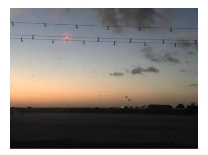
Figure 2: A power line that has been mitigated with 'bird flappers' to prevent collision
